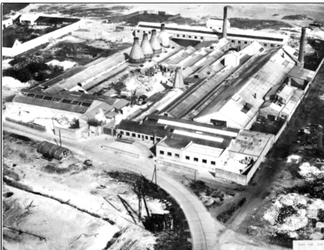
Figure A3.12: Arklow Pottery Factory c. 1950 prior to the demolition of the bottle kilns
